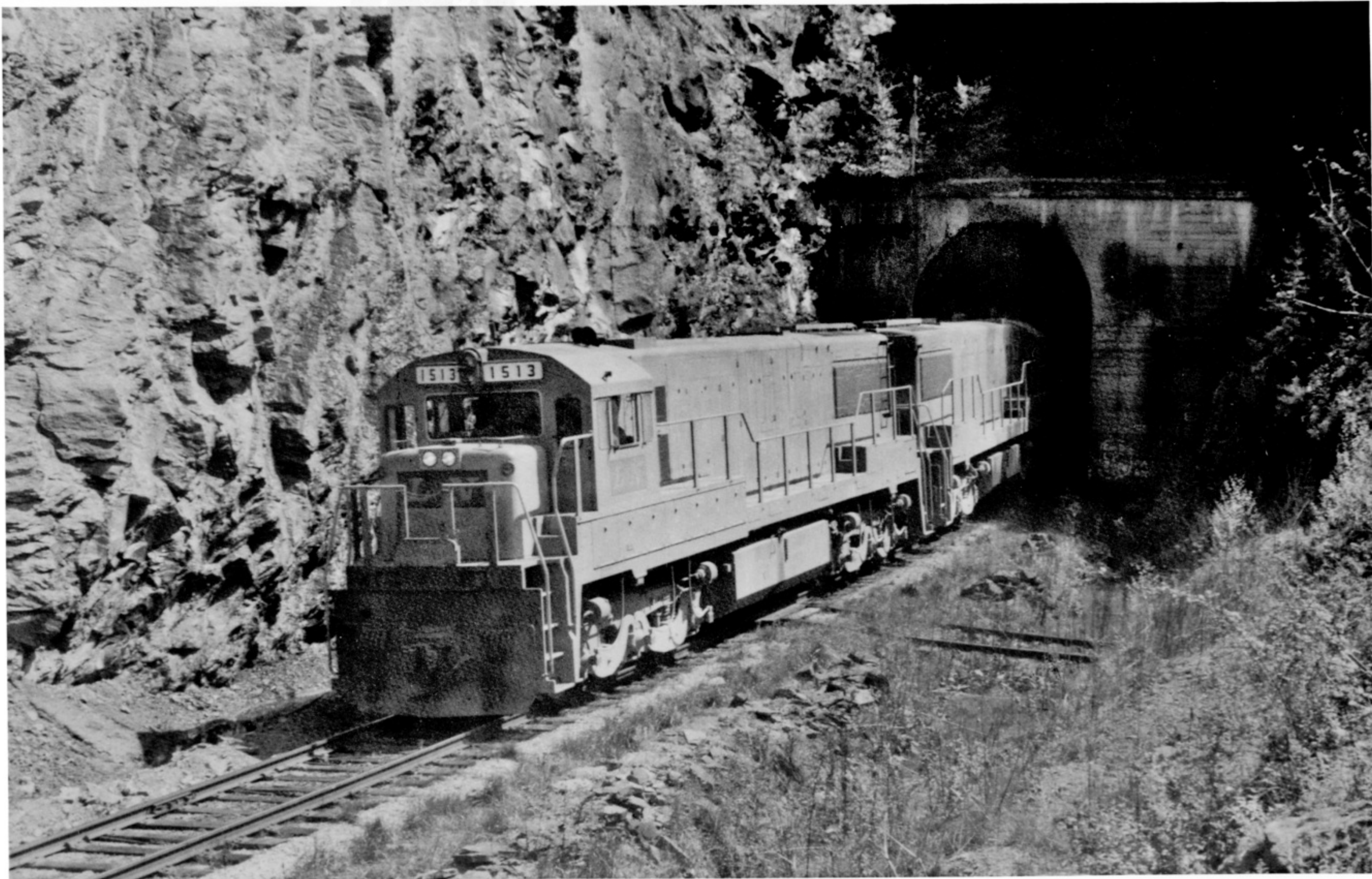
Cumberland Valley Division Fast Freight No. 66 is at the mid-point of its Norton, Virginia to Corbin, Kentucky run on a sunny summer day in 1966. Three General Electric U25Cs are shown at the north portal of 6,244-foot long Hagans Tunnel near Smith, Kentucky. This was the Old Reliable's longest tunnel, opened for service in 1930 as part of the "CC&O Connection." (Ron Flanary Photo)
