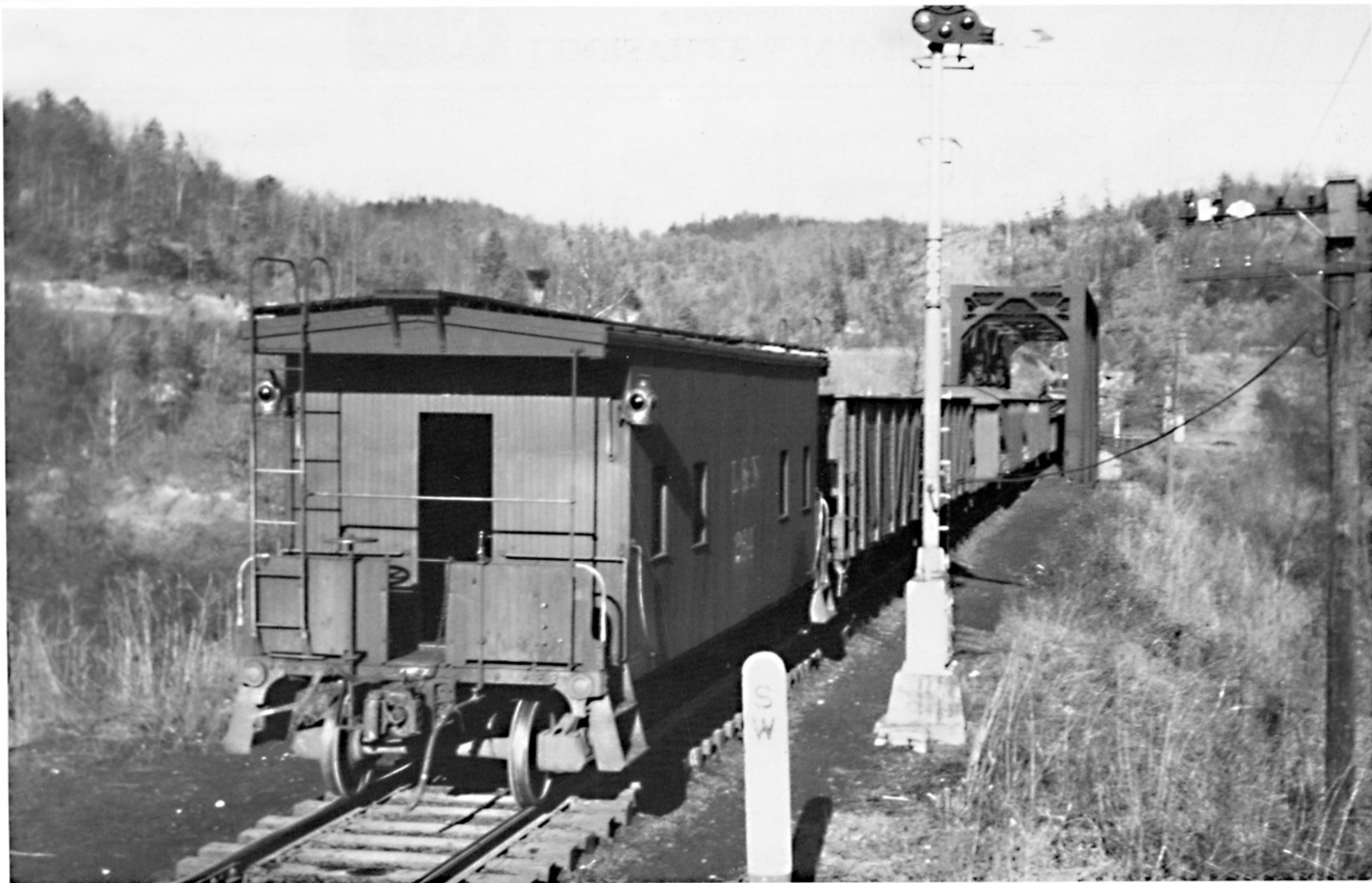
A northbound K&A Division mine run eases into Holton, Tennessee in the late '40s trailing "box car" caboose 264, one of the "sans-cupola" versions of this series. These hacks were designed for mine run, local and transfer service. (David Noble Photo/L&NHS Collection)
