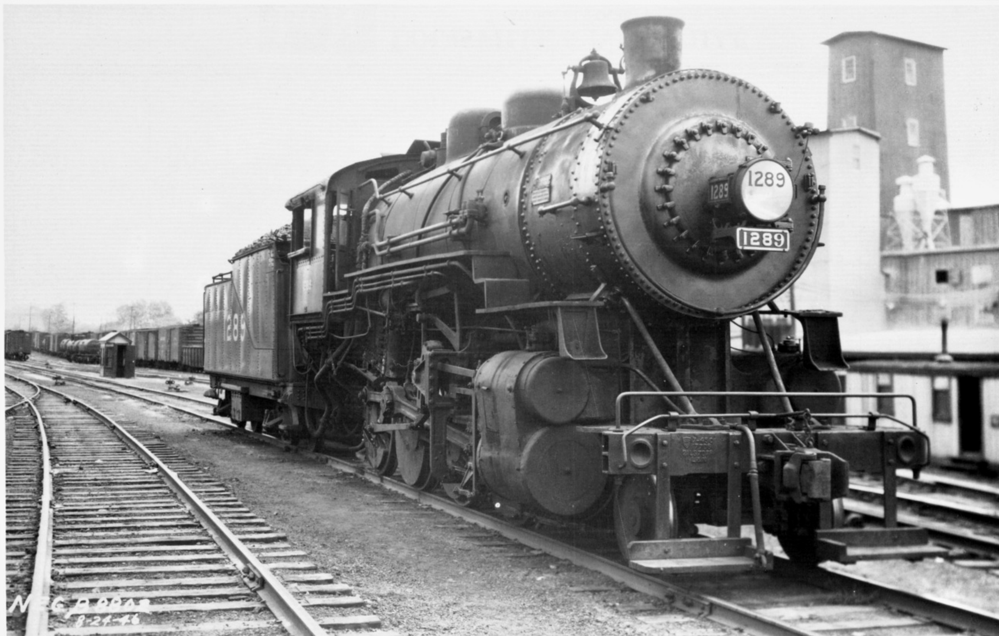
One of the 400 engines built from scratch by the L&N at South Louisville was Consolidation 1289, shown at an unidentified location on August 24, 1946. Note the unusual brass number plate, with the "128" in the more typical L&N sans-serif style, but the "9" in Railroad Roman. As with most L&N-built power, the engine has few efficiency appliances — the perfect embodiment of L&N's mechanical simplicity. (L&NHS Collection)
