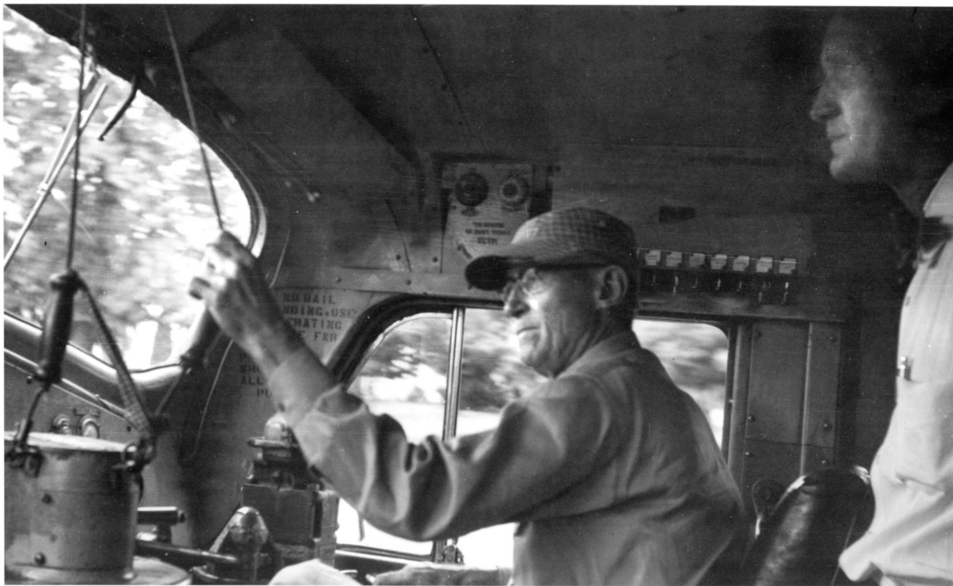
On an August day in 1959, veteran LC&L (Short Line) engineer L.A. Wells has the southbound Pan-American in full flight a few miles north of Worthville, Kentucky as Traveling Engineer Russell White observes. Note the two whistle lanyards for the E7—the low octave “country” horn, which Mr. Wells is using, and the higher pitched “city” horn, which was deemed more appropriate for urban settings. (Charles B. Castner Photo)
