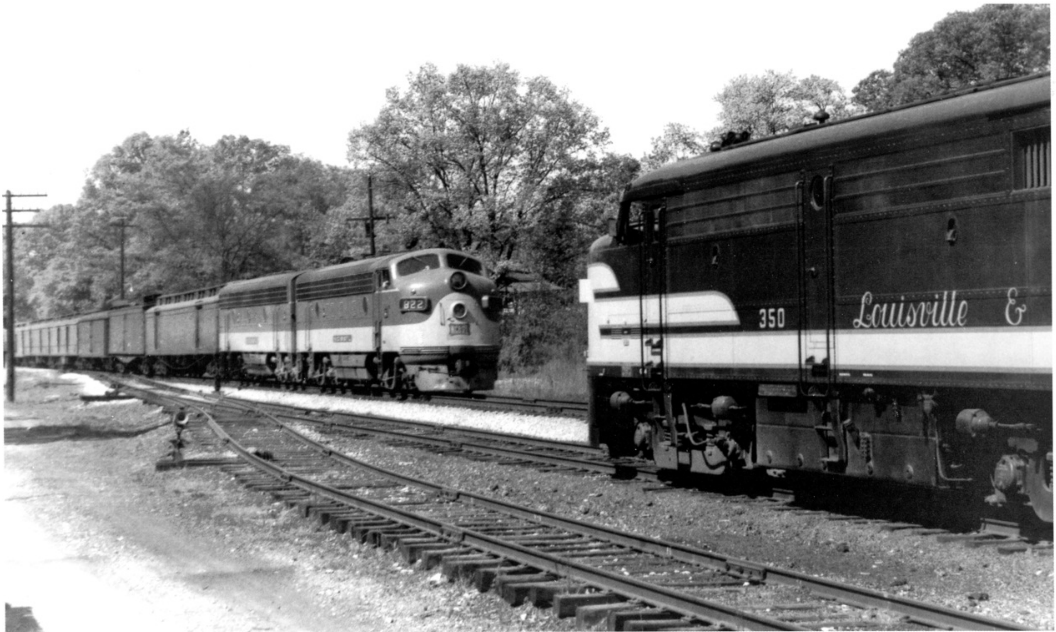
NC&StL 822 is on the point of the Dixie Flyer , train 94, at Vinings, Georgia on April 23, 1952. In the siding is an L&N extra freight led by dual-service FPA2 (which L&N classed as an FA2) 350. Note the wooden baggage car with truss rods — still common, but not what one would expect to see on a main line passenger train. (W.B. Gwaltney Photo, Charles K. Marsh, Jr. Collection)
