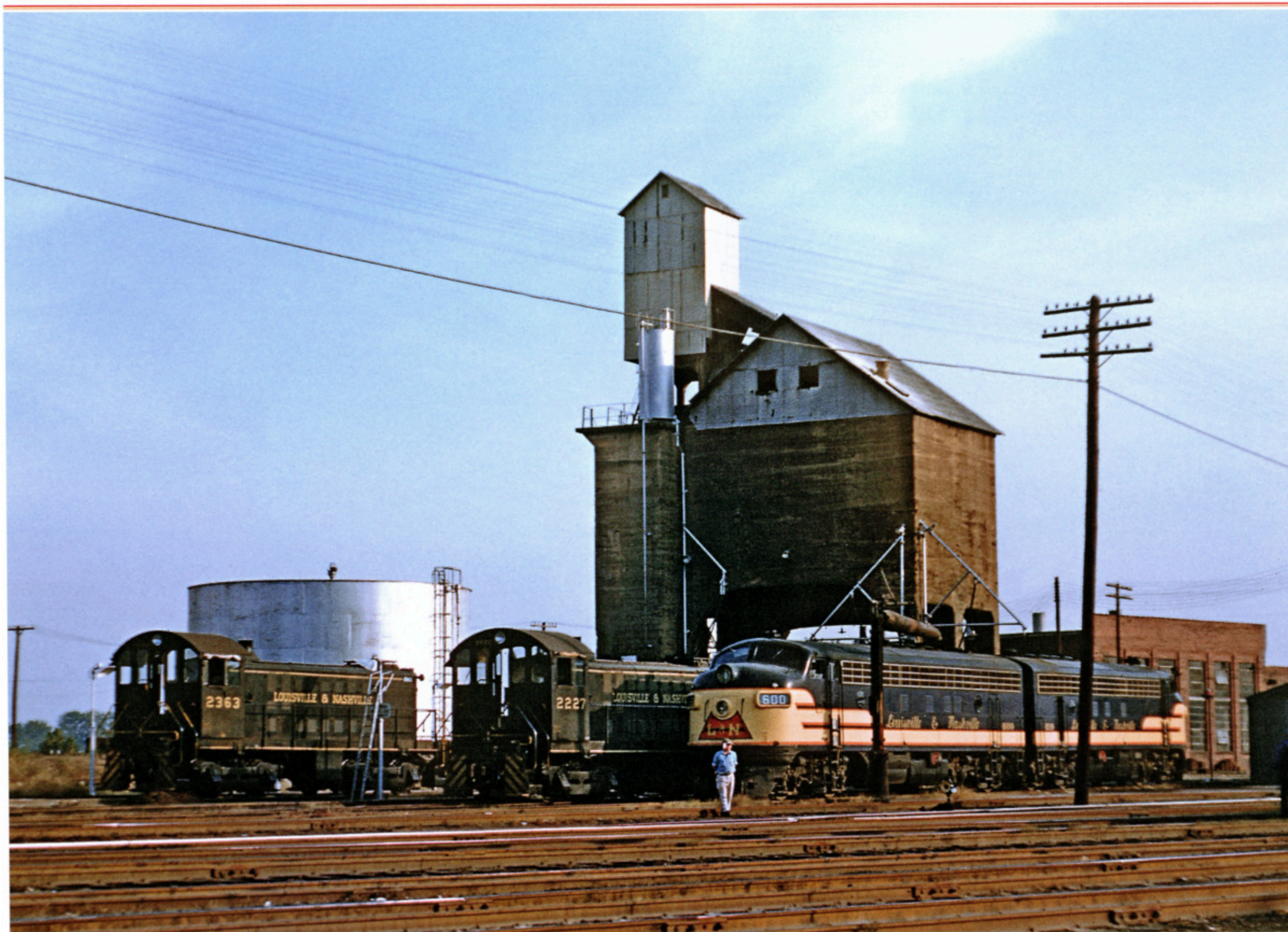
A pair of L&N FP7s off a recently arrived passenger train shares the engine house at Howell yard in Evansville on October 17, 1956 with two model Alco S4 switch engines (L&N class S-80). There were no locomotive servicing facilities at the passenger station so the cab units had to be brought to Howell yard for fuel and sand. The silver sanding system and the silver fuel tank are in service but the coal dock has not added coal to L&N steam locomotives in many years. In just 17 days, further east in Ravenna, Kentucky, the very last M-1 in service will depart with a final coal train to DeCoursey. —James Eudaly photo
